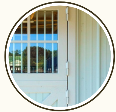
weld on hinges
