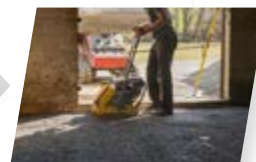
Tamp and level
